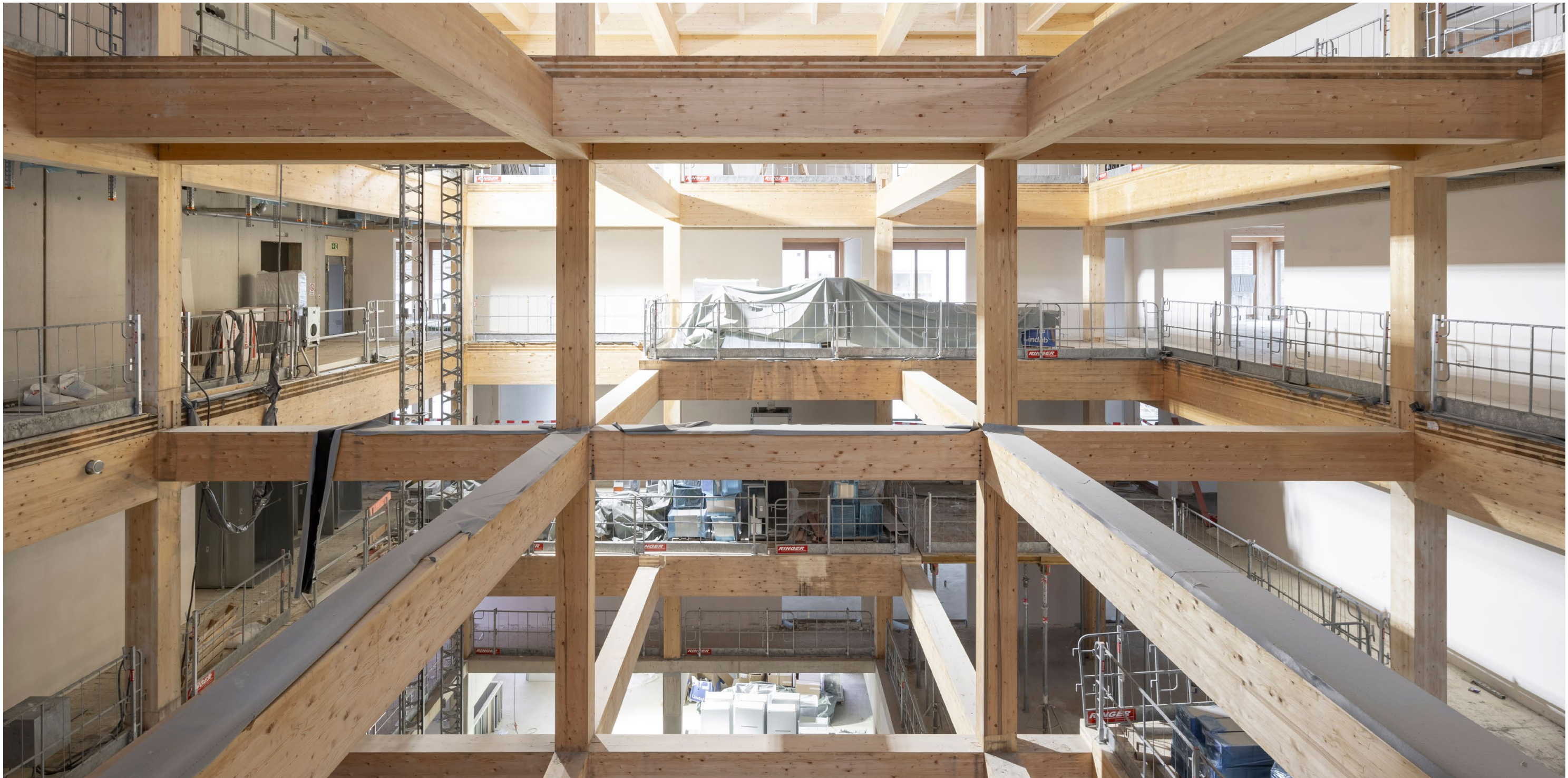
BMW Group Talent Campus, Munich – Timber-concrete composite construction, separability of the components
